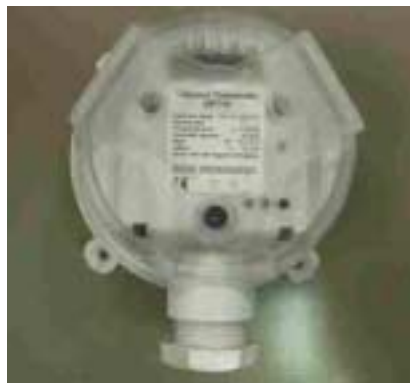
Figure 19: Room pressure switch – top view.
