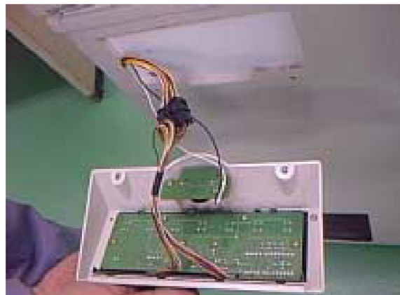
Control panel removed
