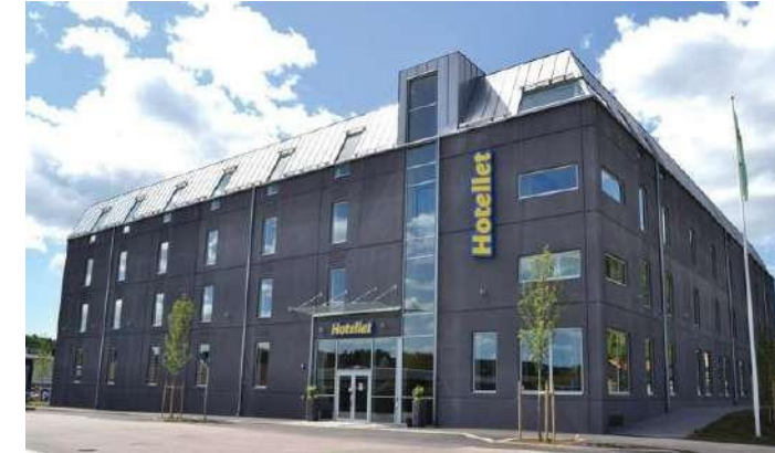
Ullared, Sweden Project: Gekas hotel Type: Hotels Product: Multilayer Plumbing System
