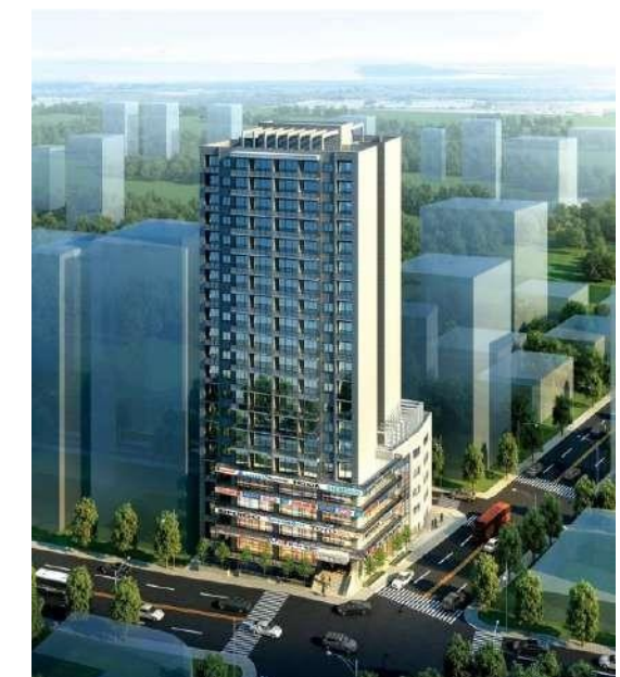
Kazanchis, Ethiopia Project: Kazadis Plaza Mix-use G+19 Building Type: Commercial Year: 2019 Product: Multilayer Plumbing System
