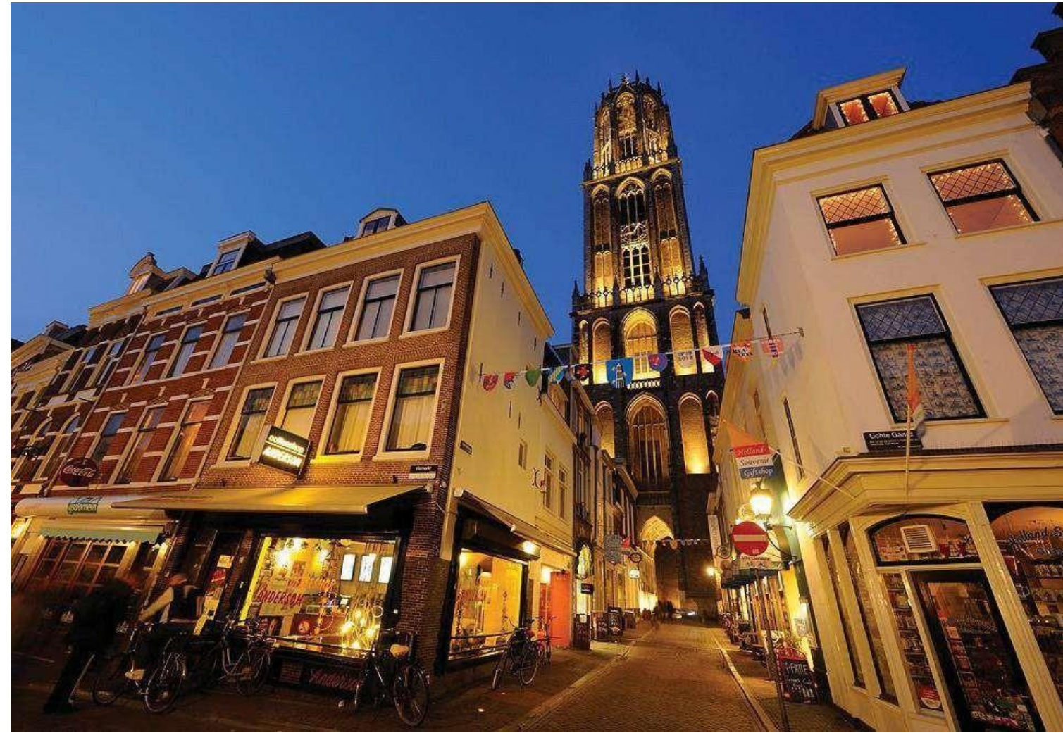
Utrecht, Netherlands Project: Domkerk Domtoren Type: Public Buildings Year: 2008 Product: Multilayer Plumbing System
