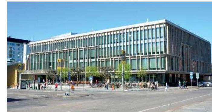
Goteborg, Sweden Project: Stadsbiblioteket Type: Public Buildings Product: Multilayer Plumbing System
