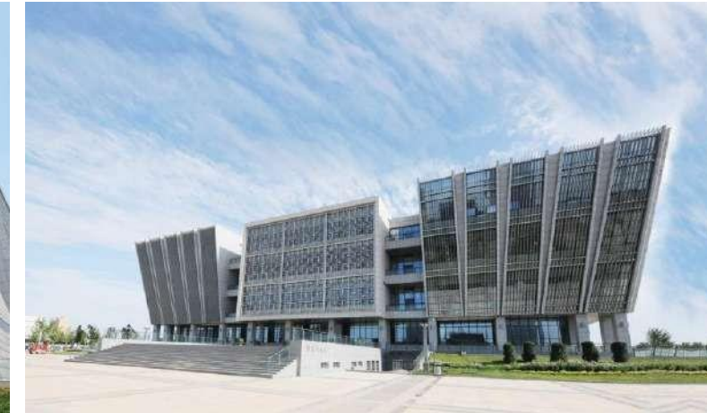
Cangzhou, China Project: Cangzhou Museum Type: Public Buildings Year: 2010 Product: PPR plumbing system
