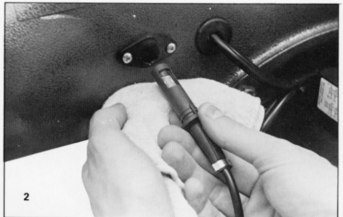
The photo cell is removed from burner for cleaning. Do not touch cell window with the fingers and use only a clean dry cloth. Ensure viewing face points towards burner combustion head when replacing.
