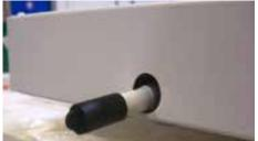
After removing the protection cover, make sure that the pipe is intact and undamaged, especially at the pipe end. Crocked or in other ways imperfect pipe ends will result in leaks. Deburr the pipe on the inside and the outside, using a deburring tool before installation
