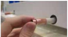
Mount a compression coupling and/or a valve to the pipe. Don't stress the nut too much, since this may crush the pipe.
