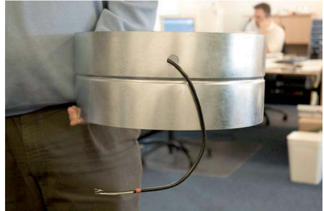
Put electric cable through drilled hole.
