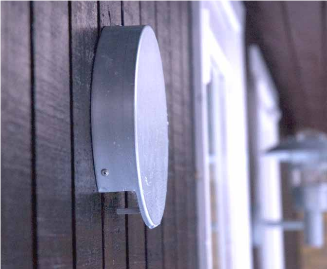
ULA, summerhouse, Dronningmoelle.
