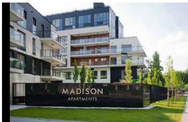
Madison Apartments - Польша - Clima Canal
