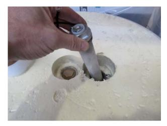
The new anode will be installed and bolted tightly. The black connection cable between the anode and the buffer must be connected again.
