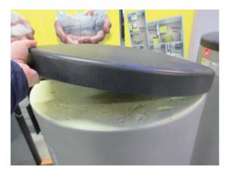
The foam, which serves as insulation in the area of the protective anode, must be removed.
