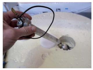
After the installation of the chain anode the drained water must be refilled. Before restarting the system, the storage tank must be checked for leaks in the area of the protection anode.
