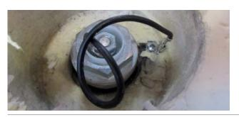
The used anode is removed by a suitable pipe wrench.
