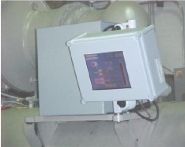
The Unit Controller and Operator Interface Touch Screen mounted on a chiller unit are shown to the left. Note that the touch screen panel is on an adjustable arm so that it can be positioned comfortably for the operator. Also note that the right side of the panel contains a built-in floppy drive from which data can be conveniently download. These are but a few of the thoughtful touches built into this control system to optimize ease of operation, reliability, and efficient operation.
