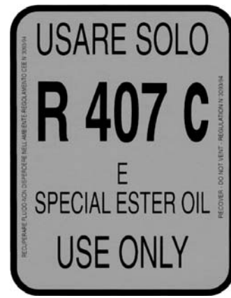
Identification of the refrigerant - External door
