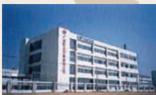
Hitachi Air Conditioning & Refrigerating, Китай
