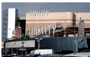
CINECITY, 12 SCREENS MULTIPLEX, SESTU, CAGLIARI - ITA
