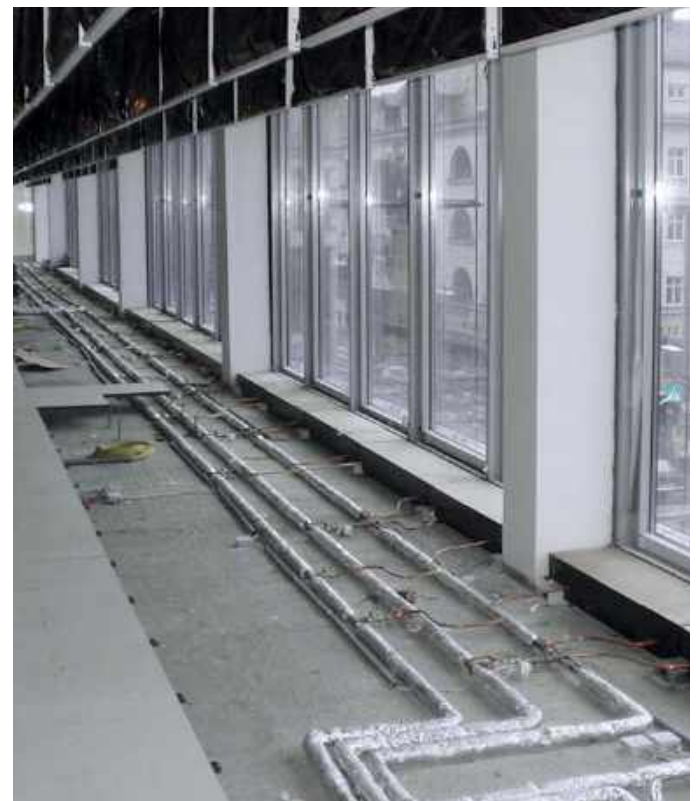
Example of double floor structure installation
