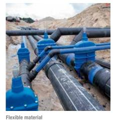
PE pipes are flexible and follow the terrain, so there is no need to level the soil in the trench.
