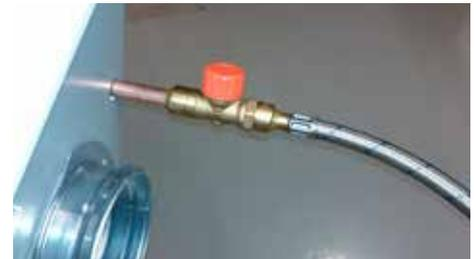
**Notice!** The connection pipes are internally soft-welded why it's not allowed to solder the beam to the pipes.
