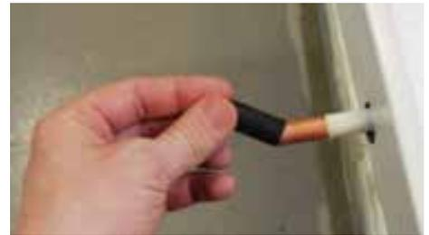
After removing the protection cover, make sure that the pipe is intact and undamaged, especially at the pipe end. Crooked or in other ways imperfect pipe ends will result in leaks. Deburr the pipe on the inside and the outside, using a deburring tool before installation
