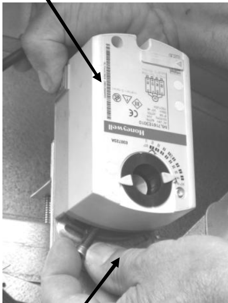
Manual rotation of the actuator
