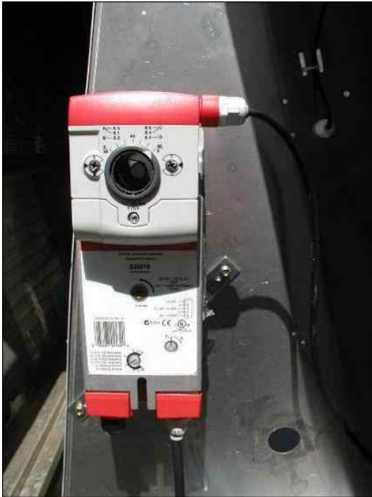
The return air damper with its auxiliary switch
