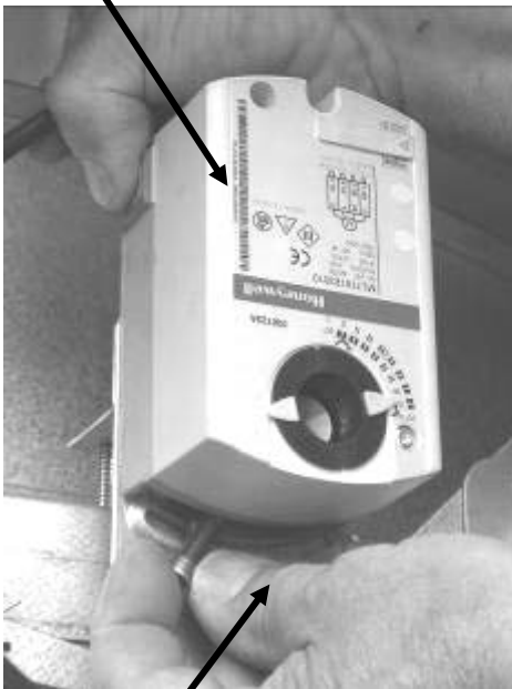
Manual rotation of the actuator
