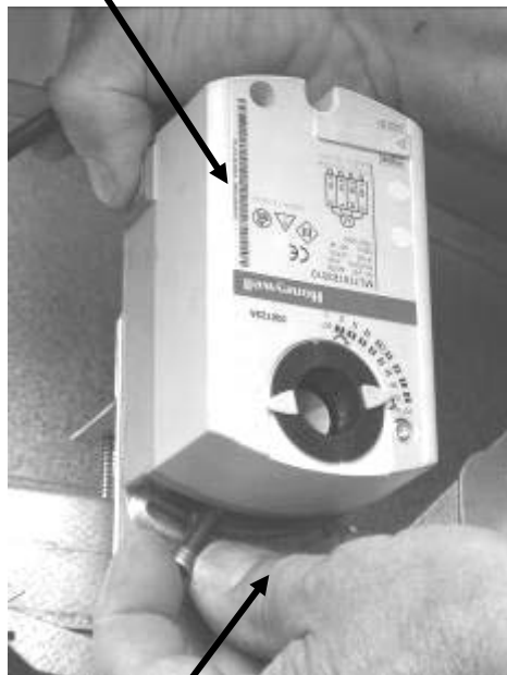
Manual rotation of the actuator
