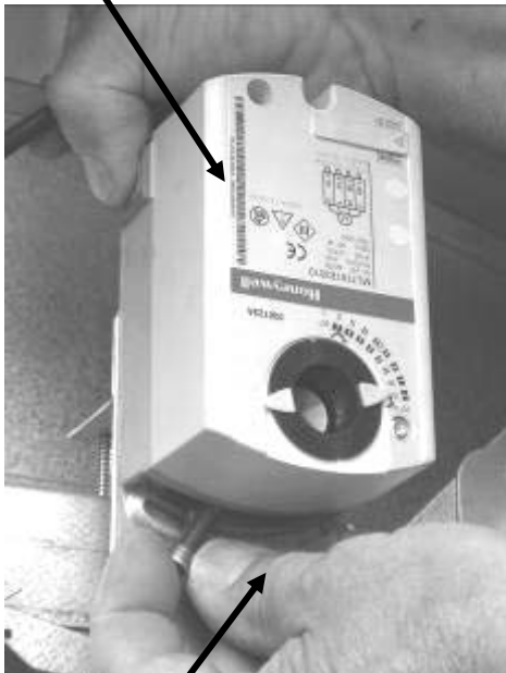
Manual rotation of the actuator
