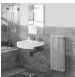
Before: Old radiator
