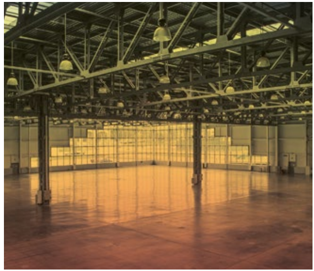
Thermography with floor heating system
