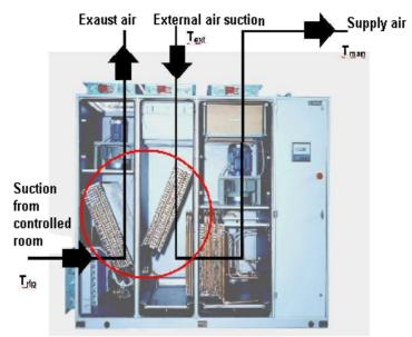
Figure 7: Heat recovery system.
