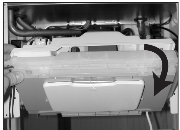
2. Tilt the boiler's electrical box
