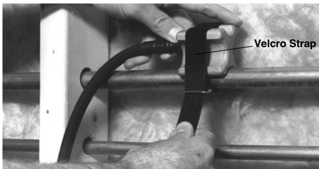
Figure 5 – Applying Freeze Head with Velcro Strap
