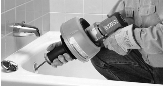
Figure 9 – Push Cable Down Drain Line
