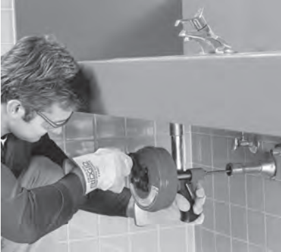
Figure 8 – Power-Spin Used By Hand
