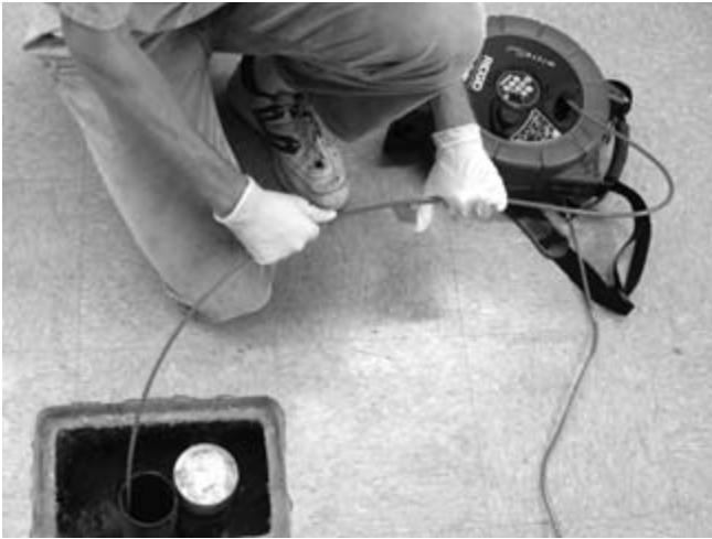
Figure 29 – Allowing cable to loop may kink the cable while pushing into drum
