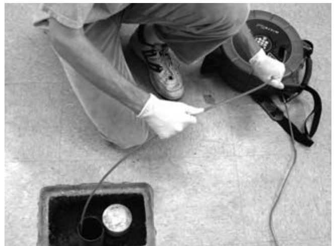
Figure 28 – Proper Technique For Pushing Cable Back Into Drum
