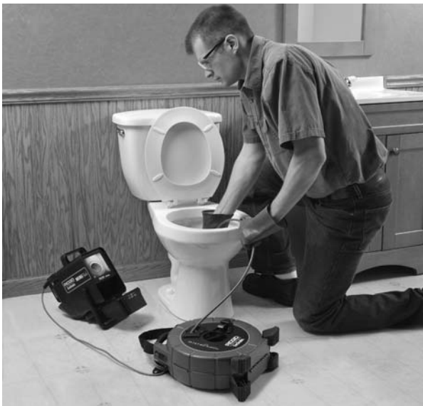
Figure 15 – Doing An Inspection
