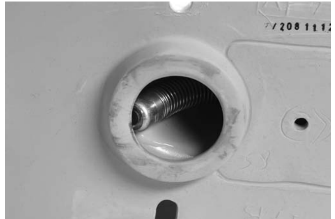
Figure 20 – Camera Head Blocked in Turn
