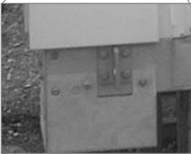
The lifting lug and the corner sheet metal have to be removed.
