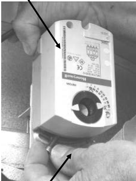
Manual rotation of the actuator
