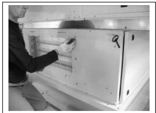
Take off the 2 hood triangle sides and the 3 last screws that will be used to fix the heat recovery support
