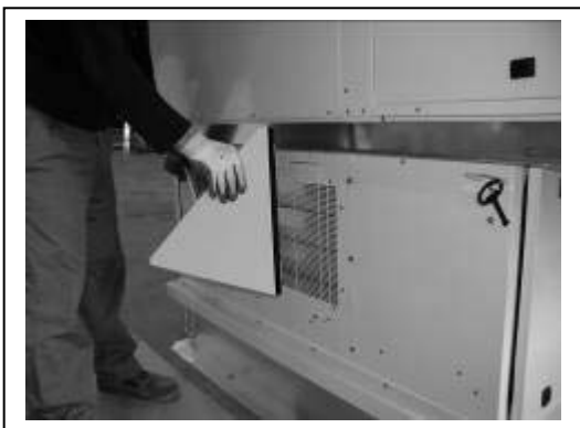
Take off the 2 hood triangle sides and the 3 last screws that will be used to fix the heat recovery support
