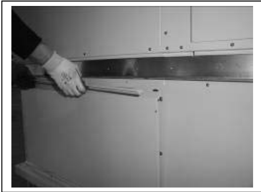
Cut the hood top angle sealant and take off the angle.
