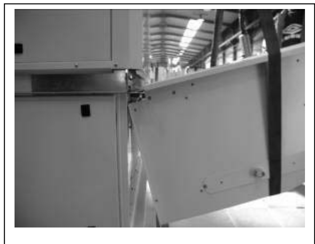
Take off the 2 hood triangle sides and the 3 last screws that will be used to fix the heat recovery support
