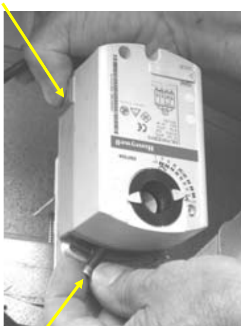
Manual rotation of the actuator
