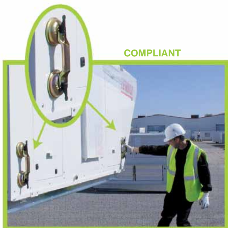
Vacuum lifting beam to position the unit
