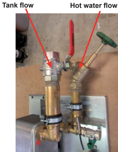
Ball valves included in the scope of delivery of the 50 l and 70 l hot water stations
