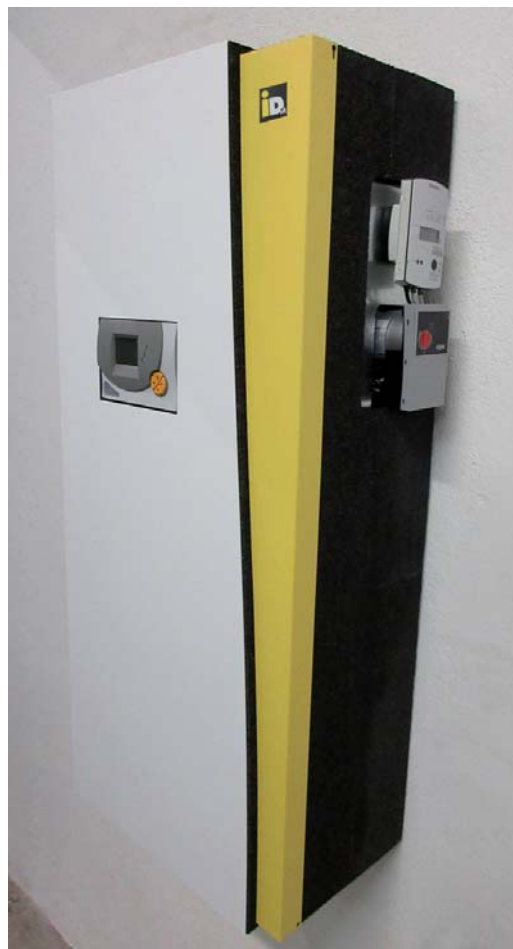
Installing the hot water station on the wall
