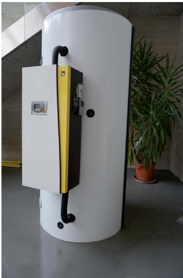
Installing the hot water station on the Hygienik
