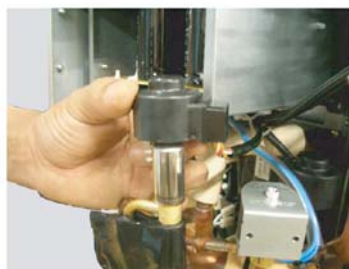
Remove the EEV coil by hand.
