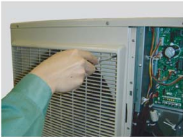
Remove the 4 mounting screws.
