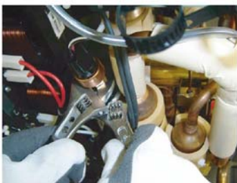
Remove the PRESSURE SENSOR with wrench.
