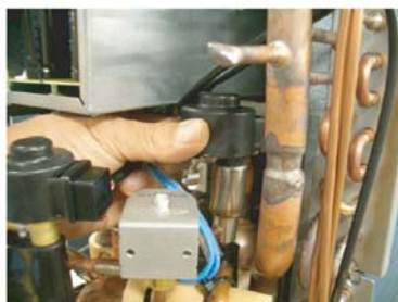
Remove the EEV coil by hand.
