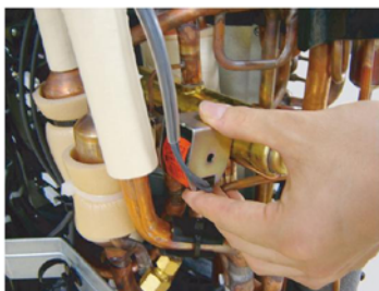
Remove the SOLENOID COIL.
