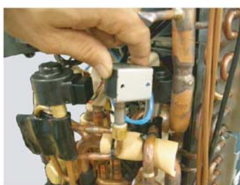
Remove the SOLENOID COIL.
