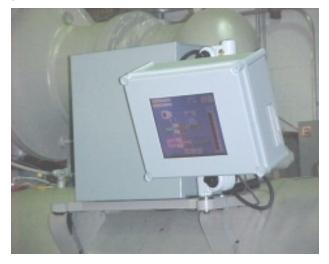
The Unit Controller and Operator Interface Touch Screen mounted on a chiller unit are shown to the left. Note that the touch screen panel is on an adjustable arm so that it can be positioned comfortably for the operator. Also note that the right side of the panel contains a built-in floppy drive from which data can be conveniently download. These are but a few of the thoughtful touches built into this control system to optimize ease of operation, reliability, and efficient operation.
