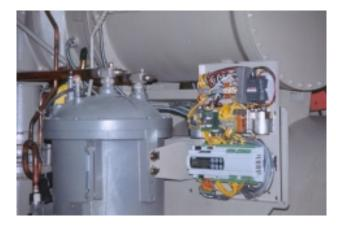
unprecedented reliability in a chiller control system. This panel also contains the oil pump contactor and overload.
