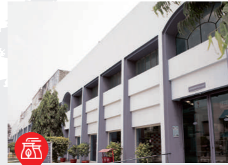
TCAI – PRODUCTION FACILITIES
