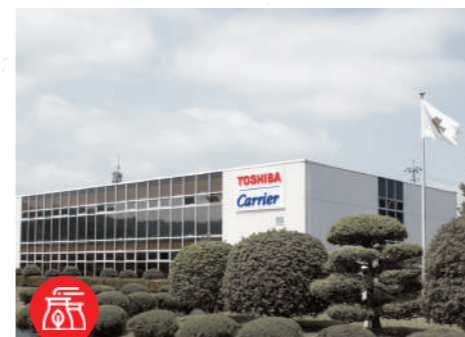
TCC – PRODUCTION FACILITIES
