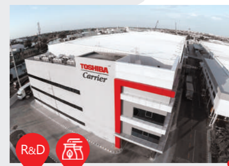
TCTC – ENGINEERING CENTRE
