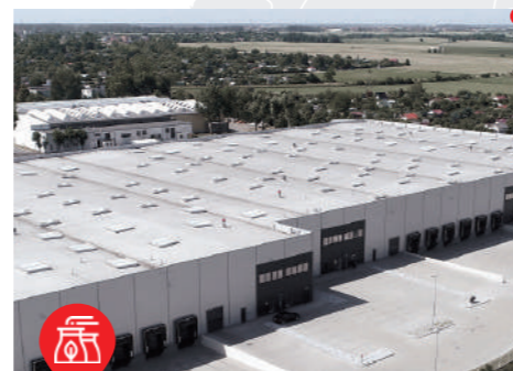
TCAE – PRODUCTION FACILITIES
