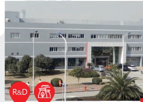
TCAC – PRODUCTION FACILITIES
