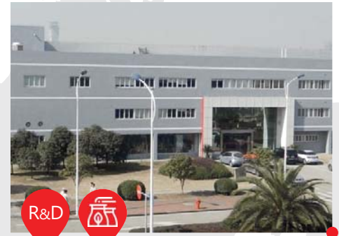
TCAC – PRODUCTION FACILITIES
