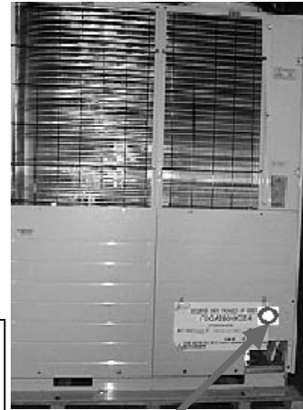
Fig. 6.11 Operation valve Open marking · Write down the time and operator of service valve opening on the surface of outside board with magic pen. · Write down the charged refrigerant amount on the inner surface of outside board
