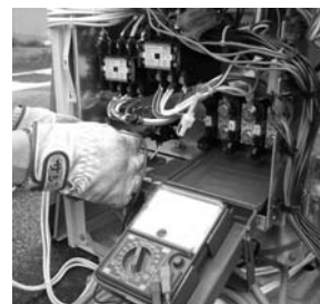
Fig. 6.9 Measuring the resistance of super link communication wire and resistance between terminal A and B
