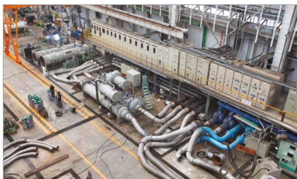
Testing platform in Korea
