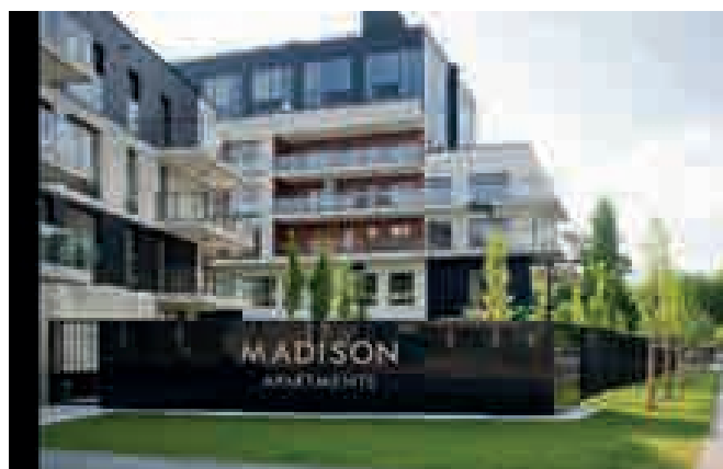
Madison Apartments - Польша - Clima Canal
