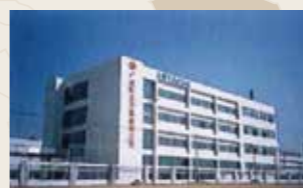
Hitachi Air Conditioning & Refrigerating, Китай
