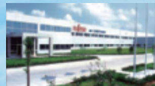
Fujitsu General (Shanghai) Co., Ltd.
