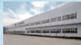
Fujitsu General Central Air-conditioner (Wuxi) Co., Ltd.
