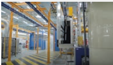
Automatic powder coating line
