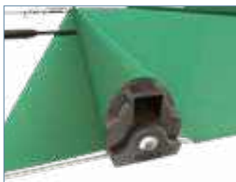
View showing the end of a cover bar with a safety and tensioning cable. The lacquered aluminium bars are the same colour as the cover material.
